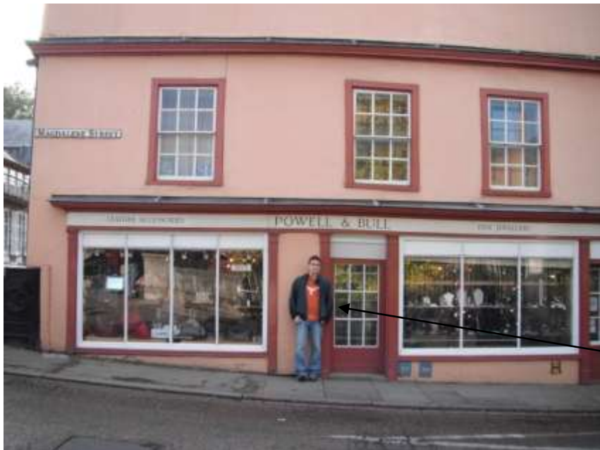
(Fig.11) Shop Front of number 26 Magdalene Street. You can see where the shop front door used to be (underneath shop sign) You can also see where the floor has been raised over time towards the bridge as the pavement is a lot closer to the edge of the window on that side than the other.
